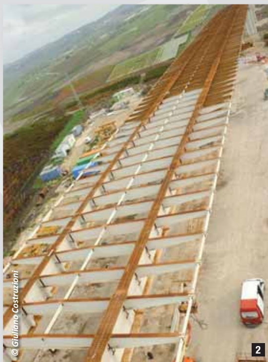
Top view of the metal deck that will support the road surface of the viaduct.
